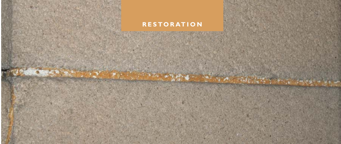
Image 1. Sydney Town Hall. Image of an early 1870s-era joint in an area of the East façade completely shaded from sunlight and the effects of weathering; as part of the original work, the off-white 'masons putty' pointing was coloured on completion by application of an iron oxide pigment. The pointing displays only minor deterioration. It is imperative that original and intact fabric in such good condition be retained undisturbed in respect for its technical heritage significance. (Image: Peter McKenzie, 4 July 2012)
