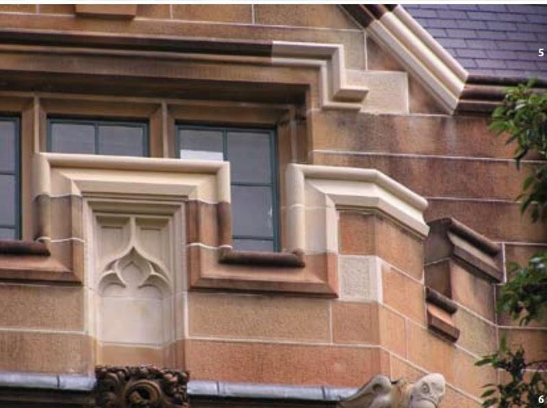
**Photo 4: Replacement stone in the parapet at the State Library of NSW. Photo 5: Wholesale replacement of stone in the pediments, tower and balustrades of Sydney Observatory. Photo 6: McCaffrey's stone in the Anderson Stuart Building, University of Sydney. (Photos: Jasper Swann, 2007)**
