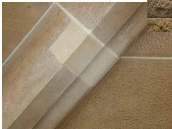
Figure 1. Small geometric indent in a raking string course. (Photo: Jasper Swann)
