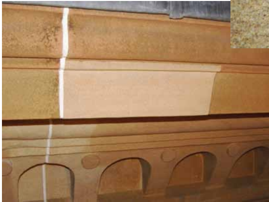
Figure 5. Hairline indent in a cornice, dovetailed at one end. (Photo: Jasper Swann).
