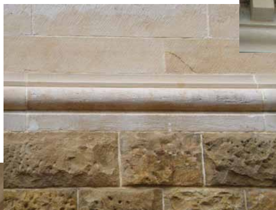
Figure 3. Indent to full length of upper moulding only of a plinth course. (Photo: Jasper Swann)
