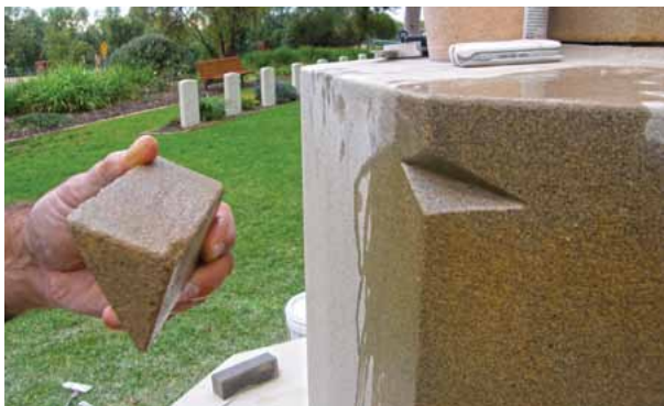
Figure 9. Damage cut away and an indent prepared.
