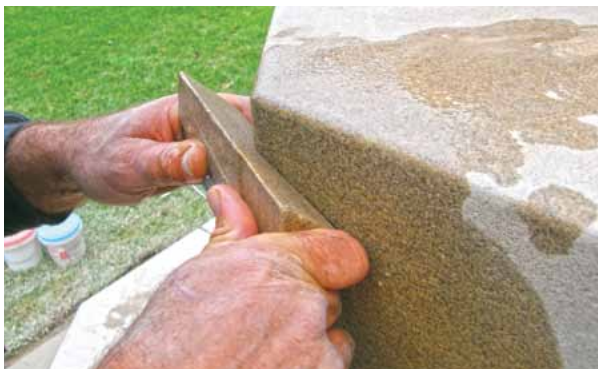
Figure 10. The indent is rubbed to a snug fit.
