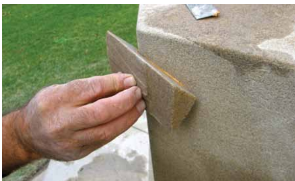
Figure 11. Indent spot-glued in preparation for dressing-in.
