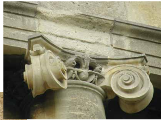
Figure 7. The missing or damaged details of this carved Ionic capital have been replaced with hairline indents. (Photo: Jasper Swann)
