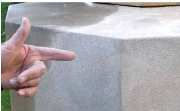
Figure 12. Repair complete. (Photos: Jasper Swann)
