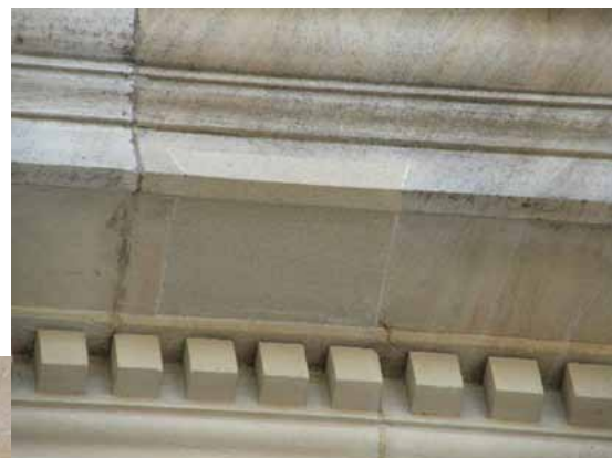
Figure 4. A well executed dovetailed indent in an overhanging element demonstrates craftsmanship and care. (Photo: Jasper Swann)
