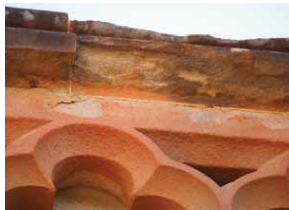
Figure 3. Failure of parapet copings leading to decay of the stonework below.
