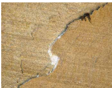
Figure 11. Cryptofluorescence, i.e. the build-up of deposited salts behind the surface of Sydney yellowblock. (Photo: Jasper Swann, 2008)
