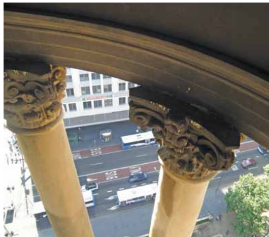
Figure 2. High above Sydney's busy George St, the ten Corinthian capitals take the load of the dome above.
