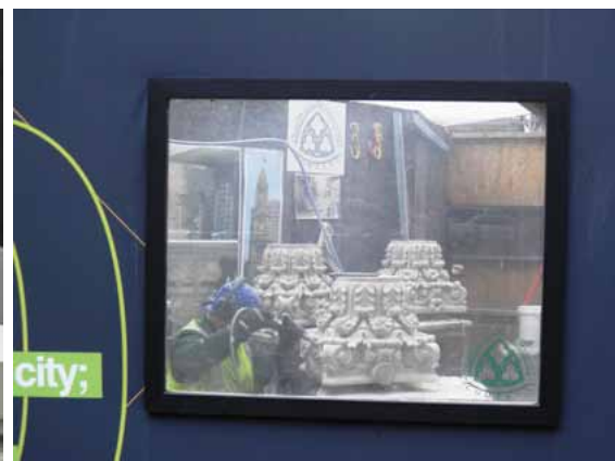
Figure 9. Window on an almost lost world. Jacek Luszczuk completes the last of the ten new capitals.
